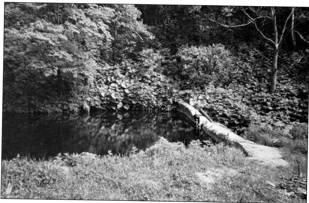
Fig. 7. Small dam in forest stream near Kostromskoye, Kholmsk District. Photo: A.N. Nilsson.
